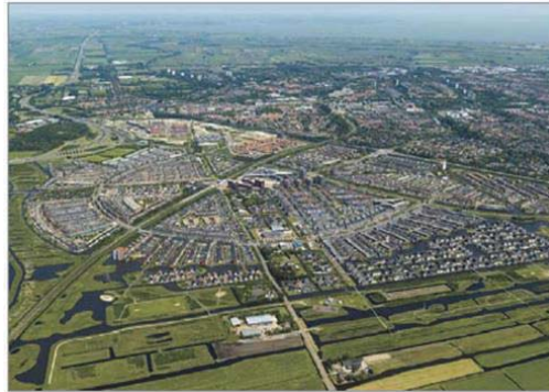
Fig. 6. Purmerend City (the Netherlands). A living example of Slim grid energy grid. Sky Pictures
