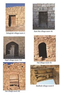
Figure 22: Examples for door opening forms and lentils types in the traditional villages in Petra region (photo: Sa'ad Twaissi & Qais Tweissi)
