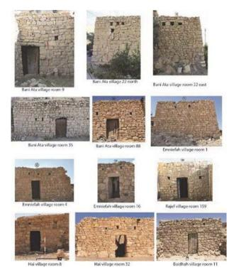
Figure 23: Examples for the forms and distribution pattern of the ventilation holes in the traditional villages in Petra region (photo: Sa'ad Twaissi)
