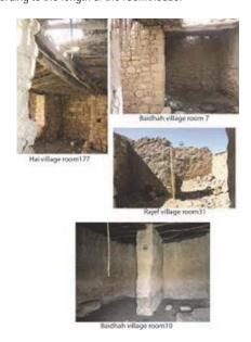
Figure 20: Examples for buttresses as roof supporter in the traditional villages in Petra region (photo: Sa'ad Twaissi
