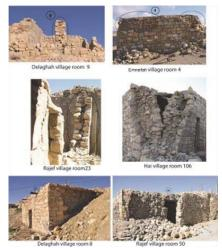
Figure 15: Examples of wall construction technique in the traditional villages in Petra region (photo: Sa'ad Twaissi & Qais Tweissi)
