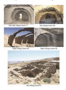
**Figure 21:** Examples for roof supported by arches in the traditional villages in Petra region (photo: Sa'ad Twaissi).
