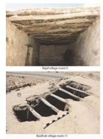
Figure 19: Examples for side walls as roof supporter in the traditional villages in Petra region (photo: Sa'ad Twaissi)
