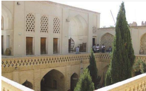
Figure 2. Pirniya House, Nain, Central Courtyard, And Source: The authors
