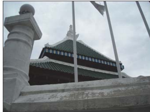
Visual 14: Kampung Keling Mosque roof structure
