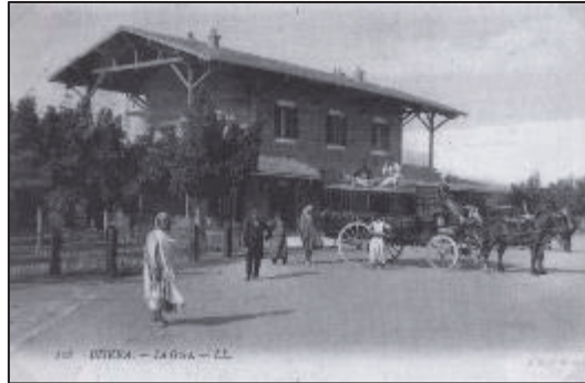
Figure 5. The Biskra railway station at the beginning of the 20th century Source: (PIZZAFERRI, 2011)
