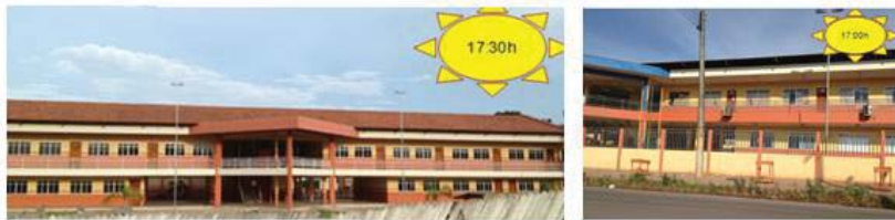
Image 08 & 09: Solar incidence on the main façade of the E.E. Profª. Nanci Nina (Aragão, 2012)
