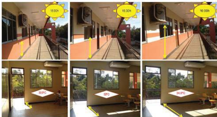
Image 07: Solar incidence on the west facade from 3pm to 4pm and penetration into the room (Aragão, 2012).
