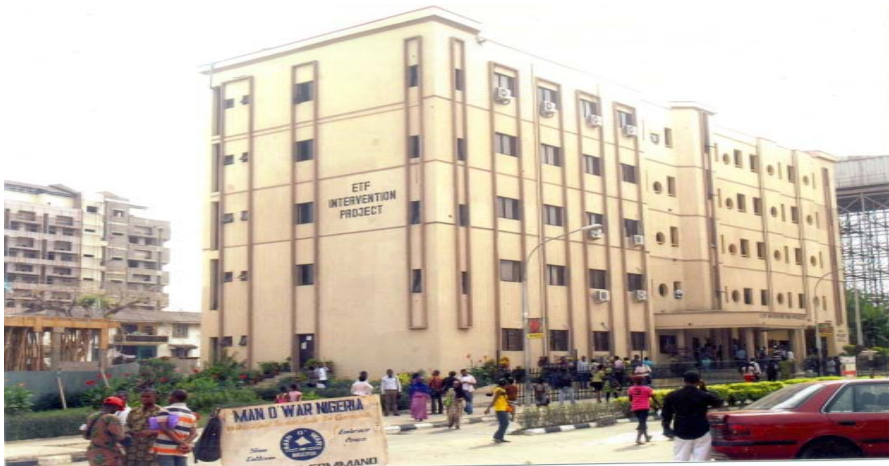
Figure 2: Completed 5 stories building named ETF building with several classrooms, lecture theater and staff offices.
