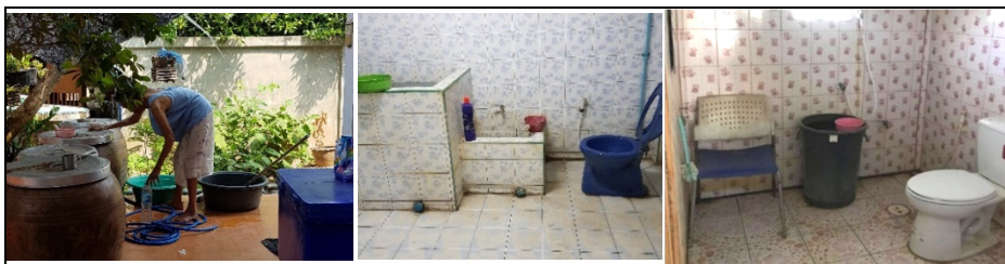
Fig 3: Some selected pictures of field activities in the study areas of bathrooms in the homes currently living by elderly
