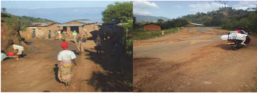
Figure 1. Condition of the Mabayi-Ruhororo road Photo 2. Condition of RN 10 Rugombo-Mabayi (Gahoma)-Kayanza
