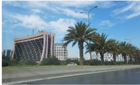
Figure 4: The Business District In Bab Ezzouar Source: Author, August 2018.
