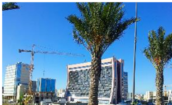
Figure 3: The Business District In Bab Ezzouar Source: google image, 2013.
