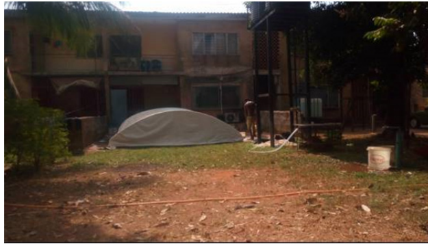
Plate 12. Showing Overhead Water Tanks which implies severe water shortage at FHA Housing Estate
