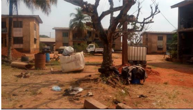
Plate 9. Showing Individual Water Tanks which implies severe water shortage at FHA Housing Estate.
