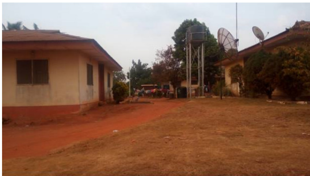
Plate 11. Showing Individual Water Tanks which implies severe water shortage at Andrew Wilson Housing Estate
