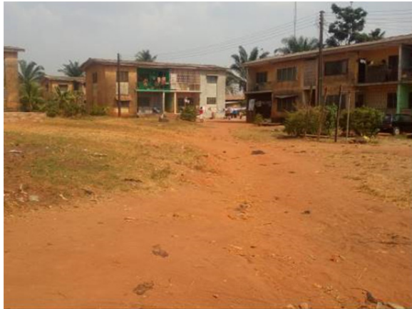
Plate 8. Showing the effect of erosion at FHA, Ikpoba Hill Housing Estate
